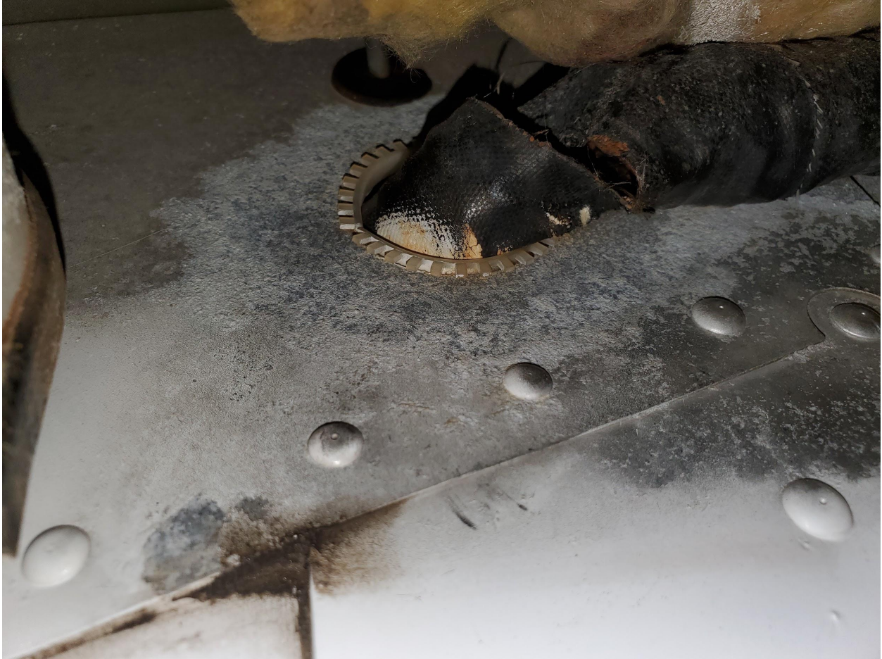
Corrosion at bulkhead (both sides similar)
